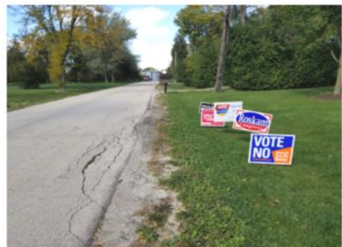
Less than 20+ feet from the roadway
